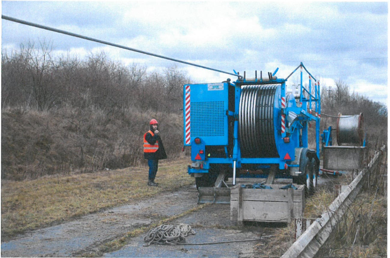
Photo 3 Stringing test arrangement
