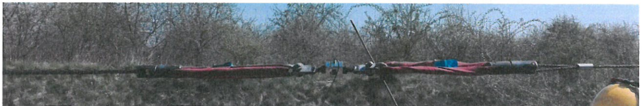
Photo 4 Pulling swivel, "Socks" and "Bug" used for stringing test
